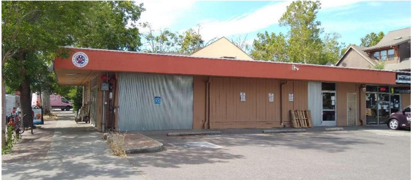
North façade (east end), ESA 2022.
