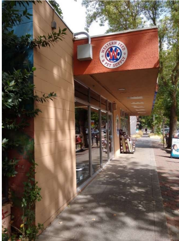
East (primary) façade, looking north. ESA 2022.
