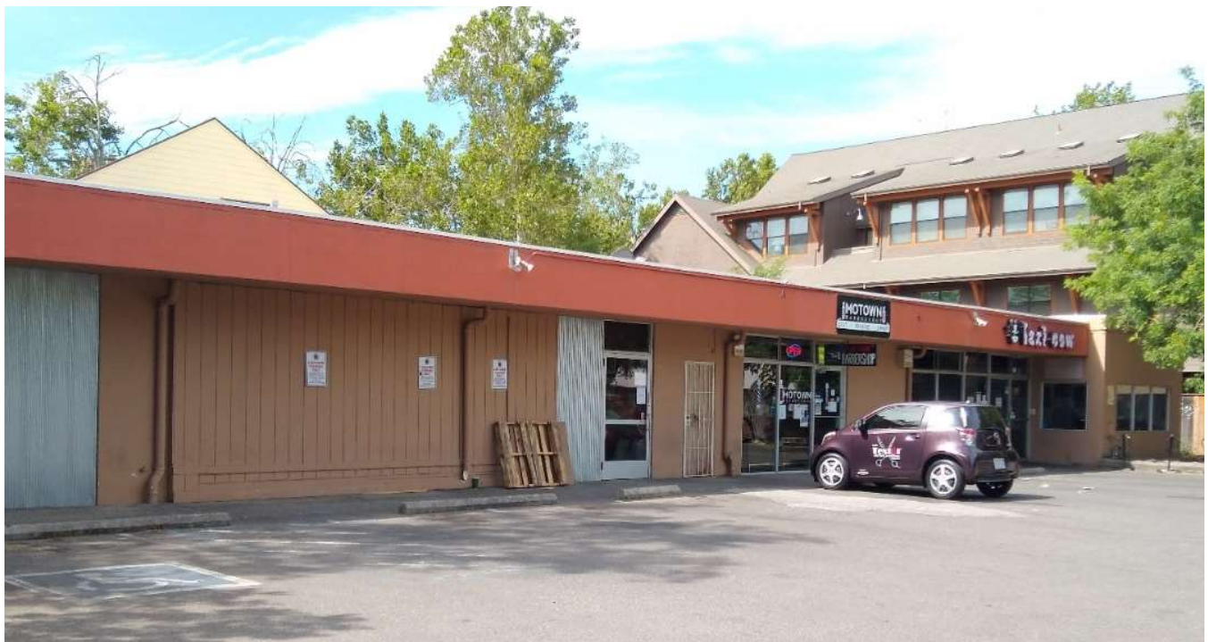
North façade (west end), ESA 2022.
